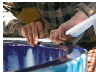
Installation of GORE® Gasket Tape Series 1000
